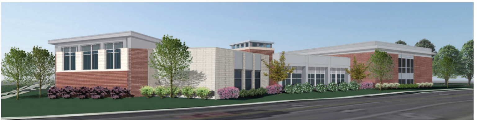
Side view from Wentzville Parkway
