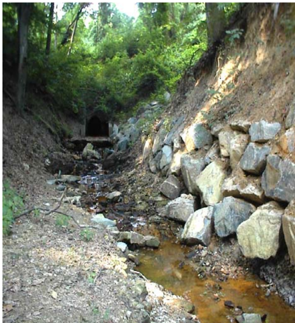
Figure 5-21 - Typical Example of Boulder Bank Stabilization
