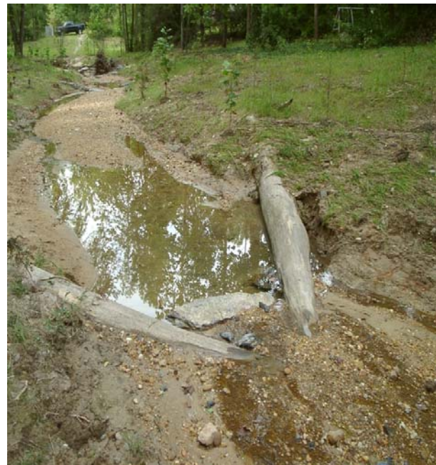
Figure 5-17 - Typical Example of a Log Vane
