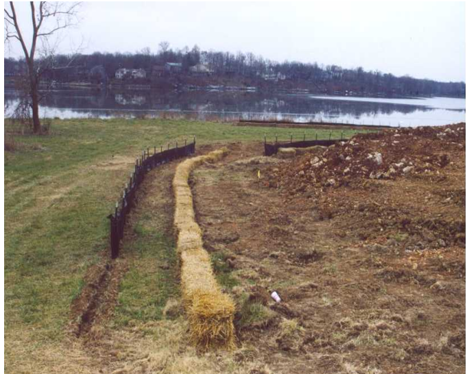
Figure 4-2 - Erosion Control at St. Joseph Hospital in Lake Saint Louis
