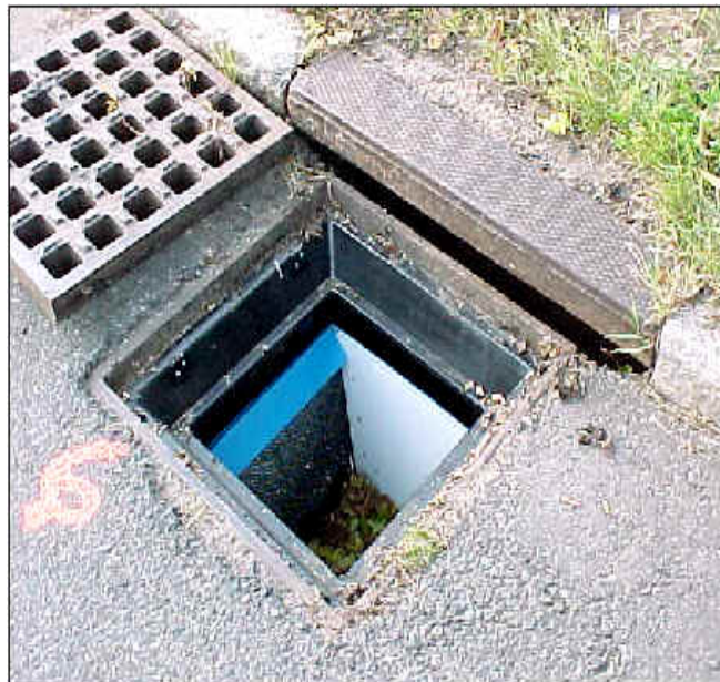
Figure 5-7 - Typical Storm Inlet Filter
