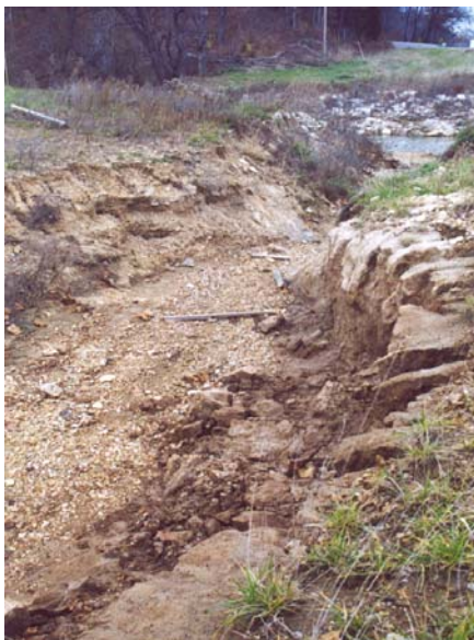
Figure 2-4 - Erosion from Discharge to Peruque Creek at Hepperman Road
