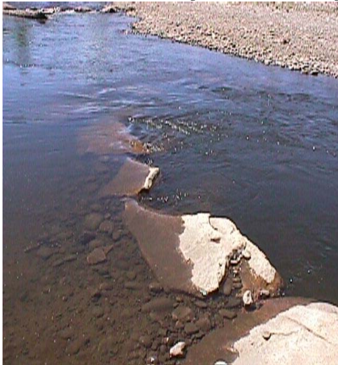
Figure 5-18 - Typical J-Hook Vane
