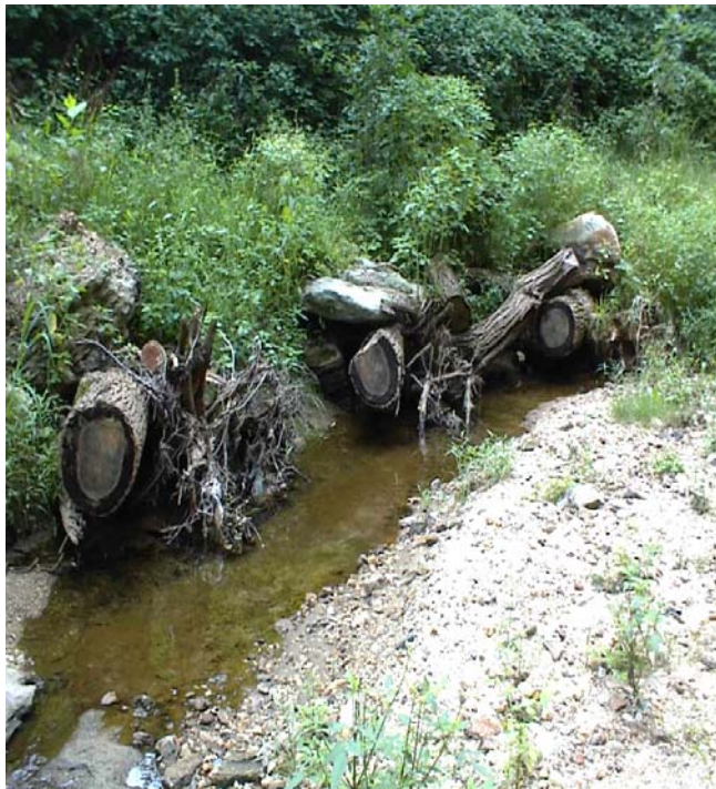
Figure 5-16 - Root Wad Channel Stabilization
