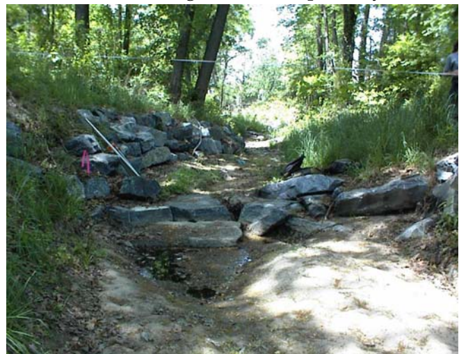
Figure 5-19 - Typical Rock Cross Vane
